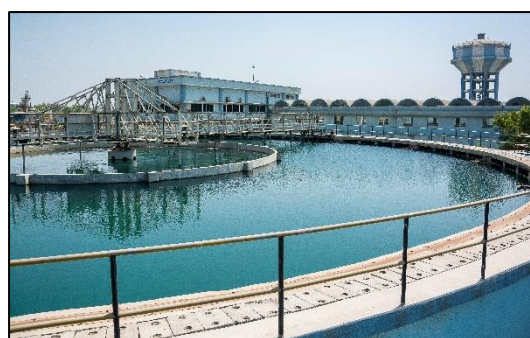
Figure 2-1: Kosad Waterworks site
