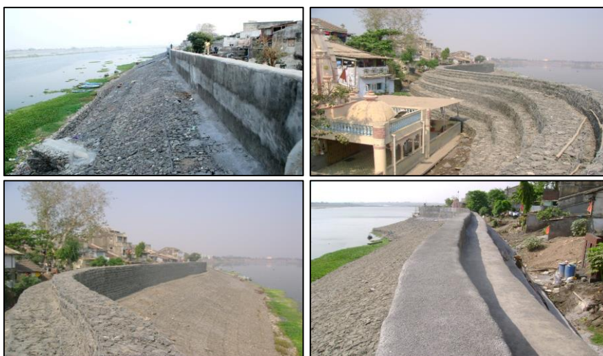
Figure 5-4: Flood protection along Tapi river
