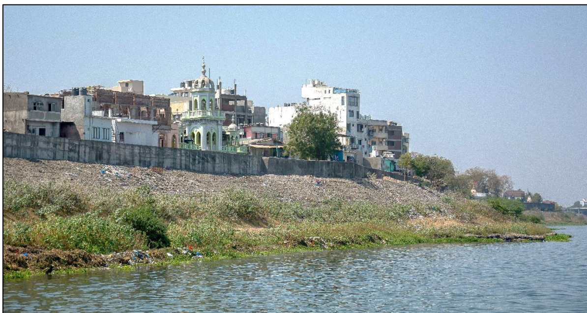
Figure 2-6: Flood protection wall near Weir cum Causeway
