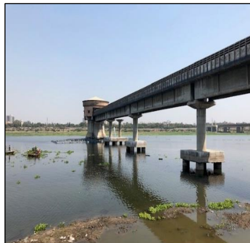
Figure 3-1: Intake Tapi River water for Katargam drinking water treatment plant
