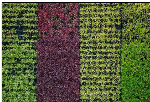
Figure 6-3: Green wall at Science Centre
