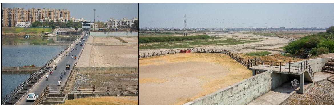
Figure 5-7: Weir cum Causeway
