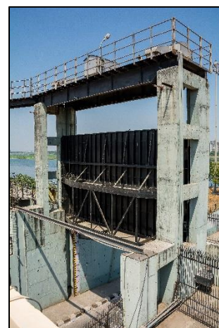
Figure 2-3: Northern gate in Weir cum Causeway
