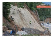
surface erosion. A biotic soil media will then be applied to enable vegetation growth. The location of the parent rock and the slide mass interface will be filled to prevent sub-surface accumulation of water. This initiative has prevented the sliding of the slope and, at the same time, the greening of the areas through the development of medium enabling vegetation growth.
