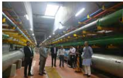
Underground Utility Tunnel (7.6m x 6.2 m) for transport
