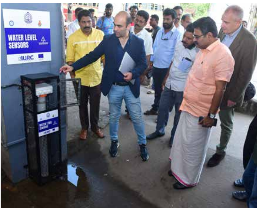
Water Level Sensors installed in Kochi
