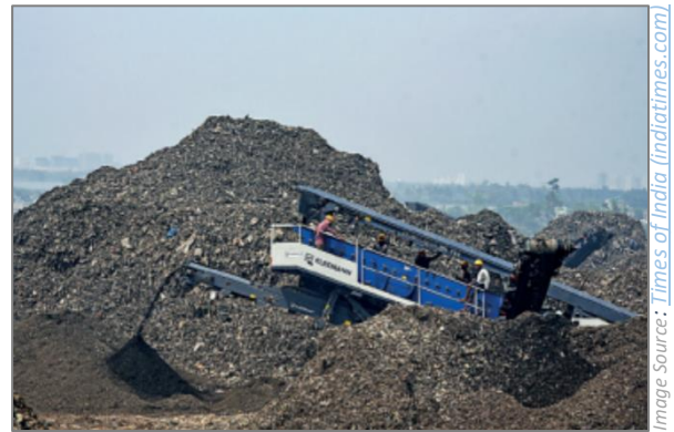
Photograph 2: Bio-mining at Dhapa
