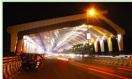
Night view of Akota Solar Panel Bridge
