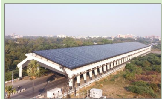
Akota Solar Panel Bridge
