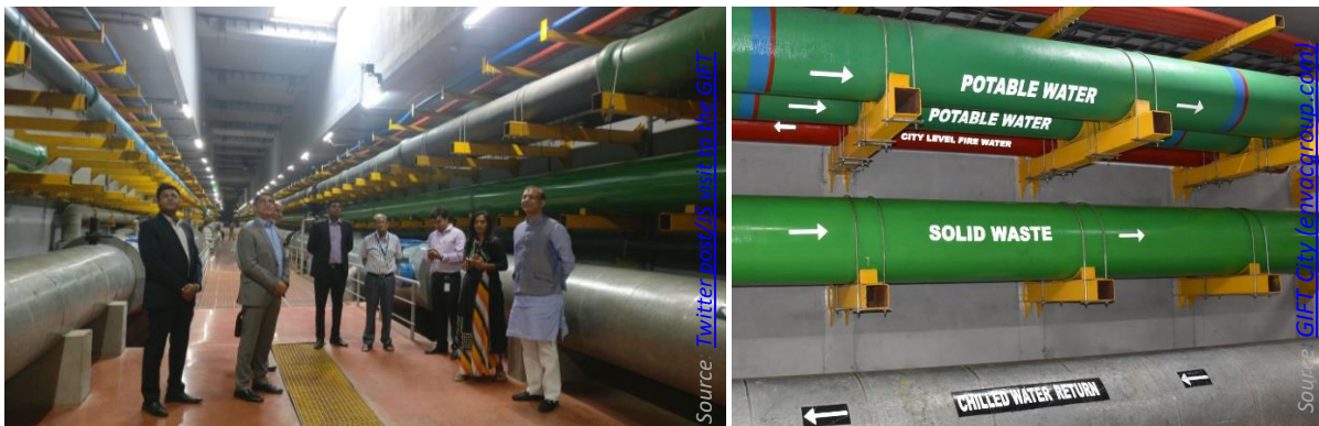
Photograph 3 Underground utility Tunnel (7.6m x 6.2 m) for transport
