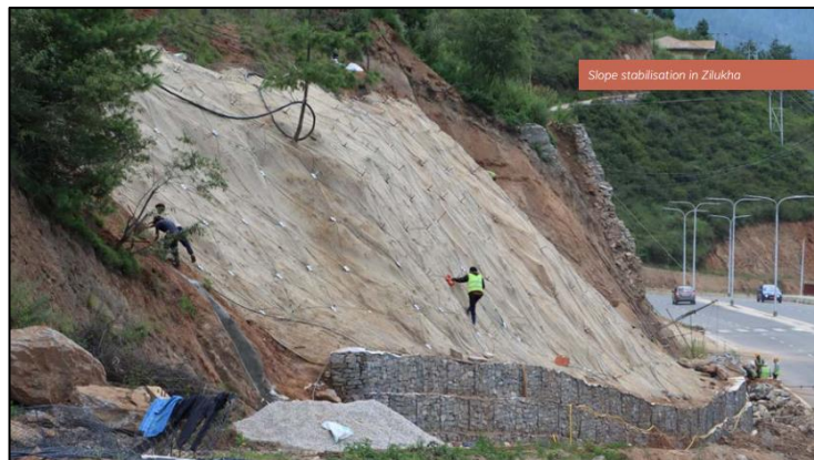
Photograph 6: Slope Stabilization in Zilukha
