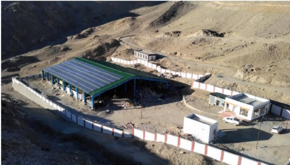
Photograph 1 Solar Powered Waste Management Facility – Leh
