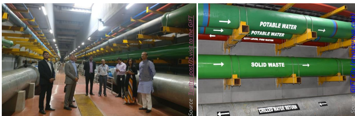
Photograph 3 Underground utility Tunnel (7.6m x 6.2 m) for transport
